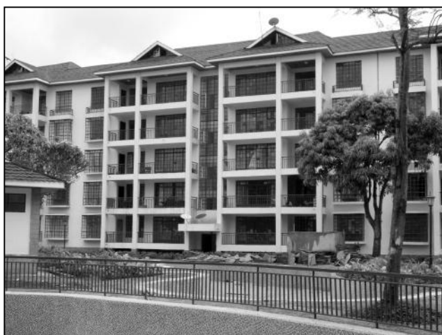
Figure 3: Picture of one building and the swimming pool of 'Jacaranda Gardens'
